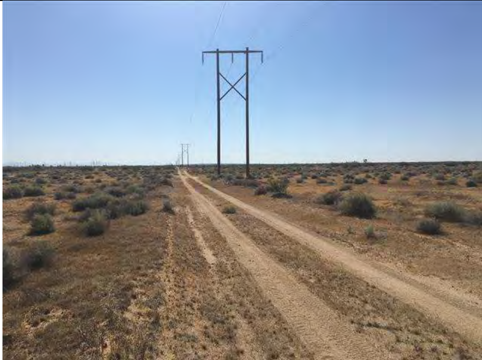
Photo #13 Facing east toward the Property alignment (Figure 6).
