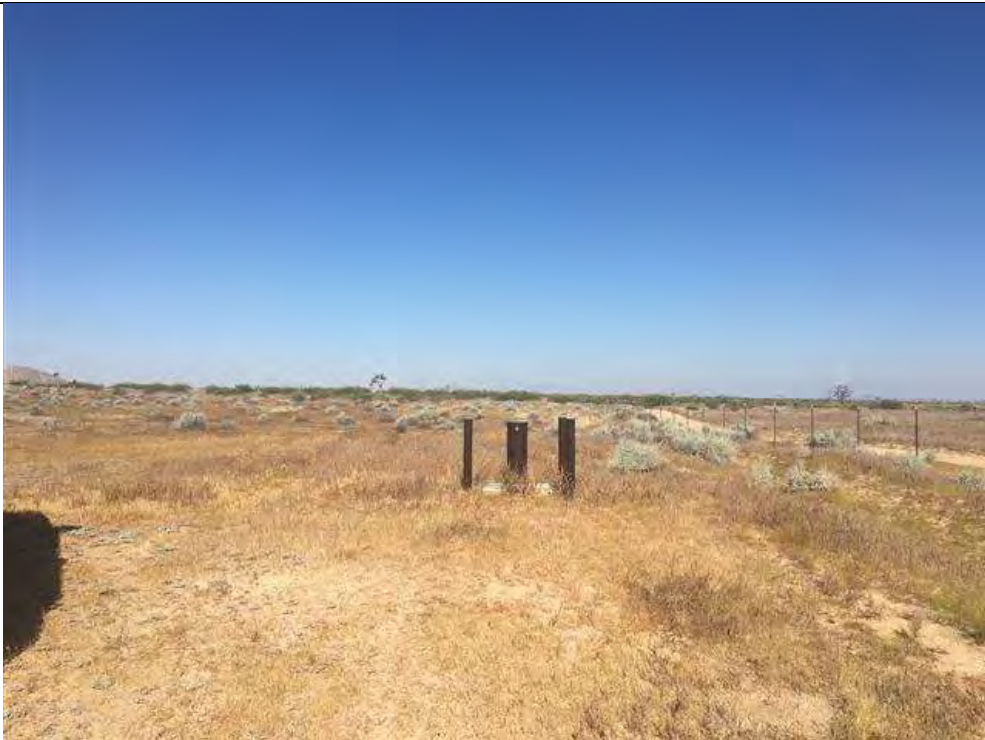
Photo #4 Facing west at a groundwater monitoring well located in the western portion of the Property (Figure 3).
