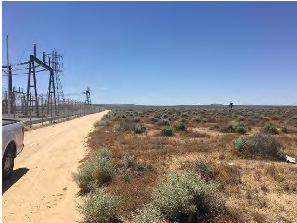
Photo #22 Facing south near the SCE Kramer substation (Figure 7).
